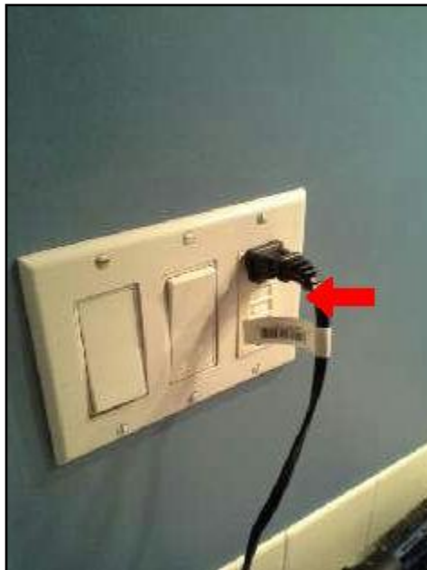
15. GFCI - bathroom
